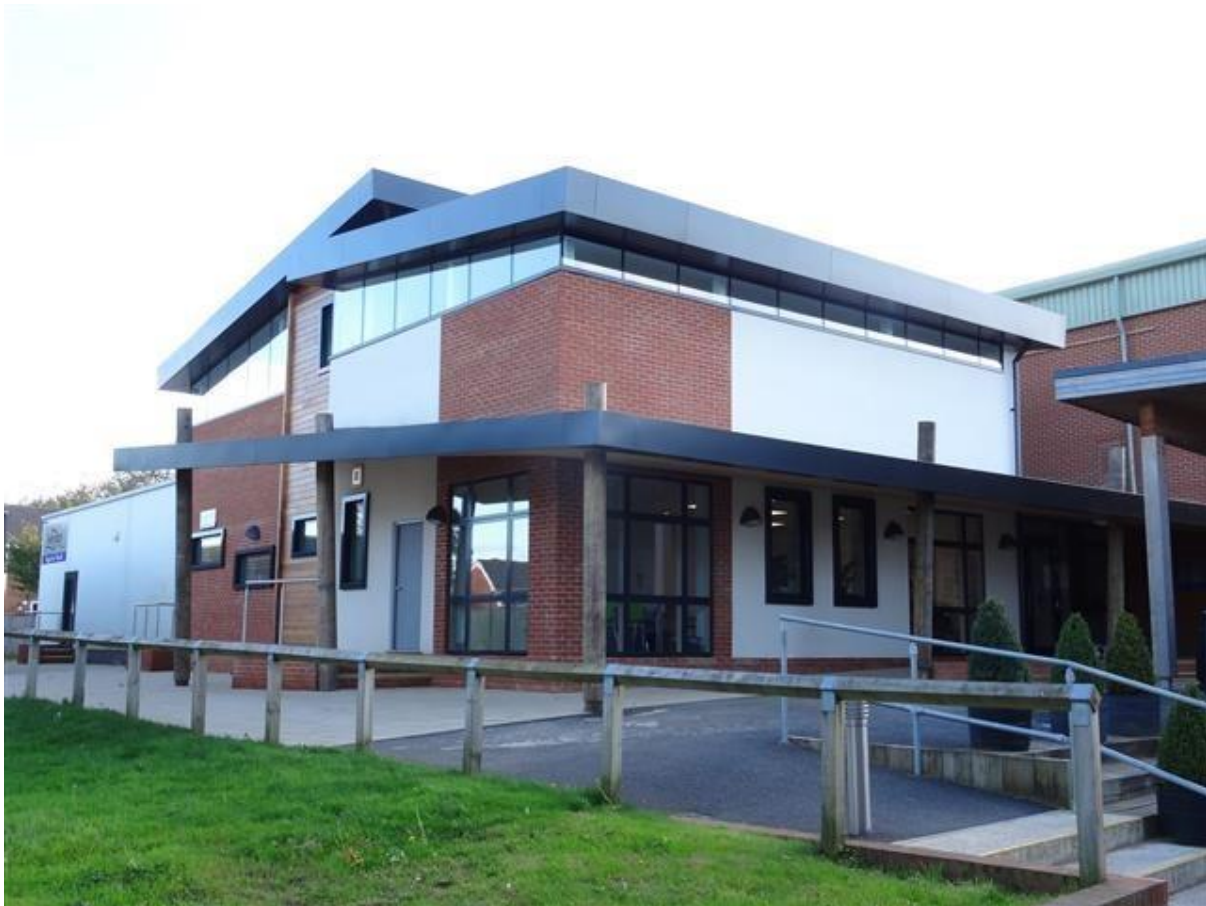
Weydon Sports Hall Extension
