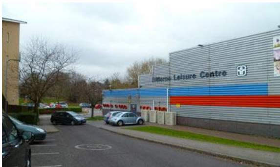
SASH Exterior Bitterne LC Southampton
