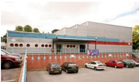
Clifton Hill L.C. SASH - Note the scale of the plinth.
